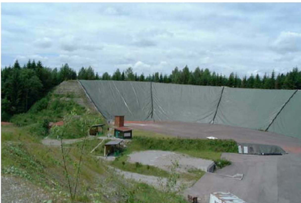
Figure 1-8: Example of a range with both a horizontal and vertical barrier (Bavarian StMLU, 2003)
