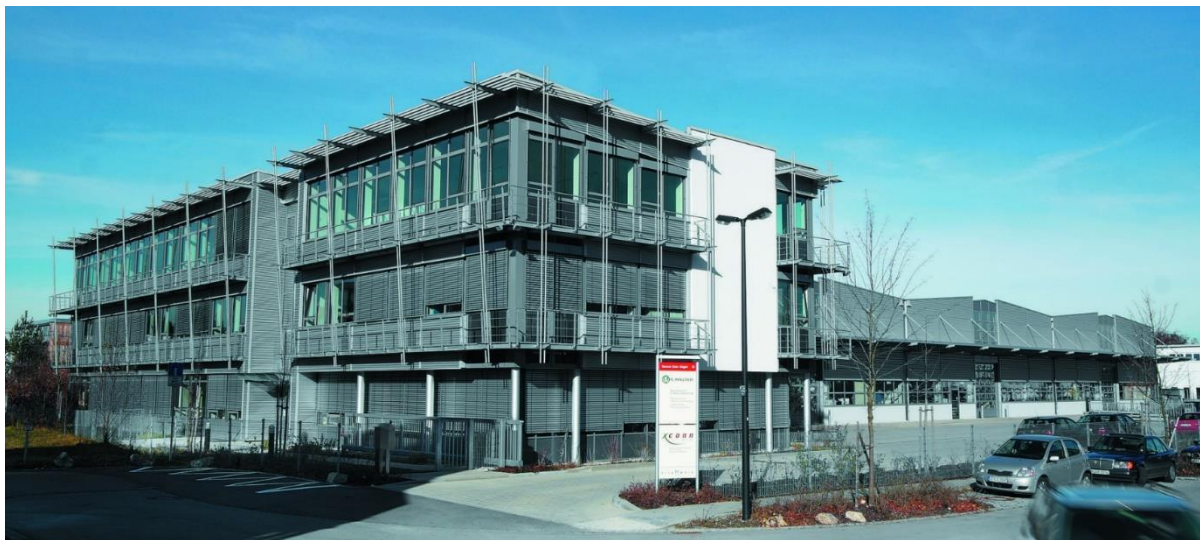
Figure 4: K. Walter’s site in Krailling
